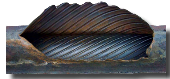
Catastrophic Rupture of a Waterwall Tube
